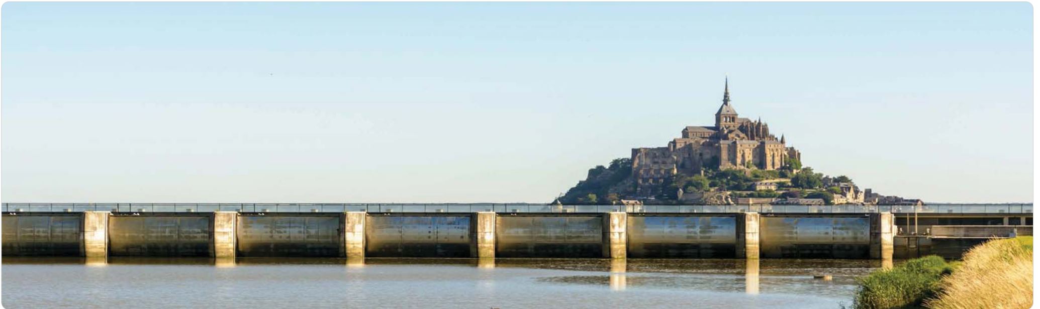
Sluice gates at the Mont Saint Michel in France
